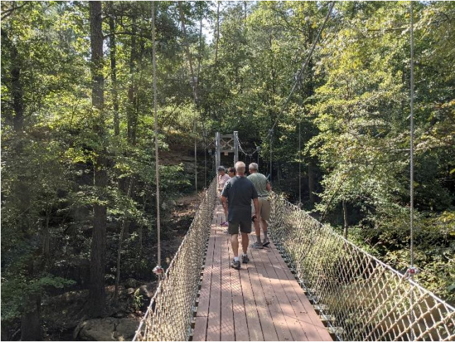
“the” suspension bridge over the Black Creek
